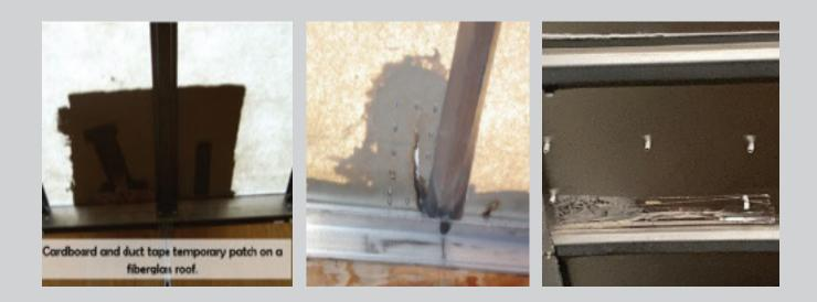
Check the tops of rolls and floor under patches or damaged areas to make sure water didn't leak through the repairs.
